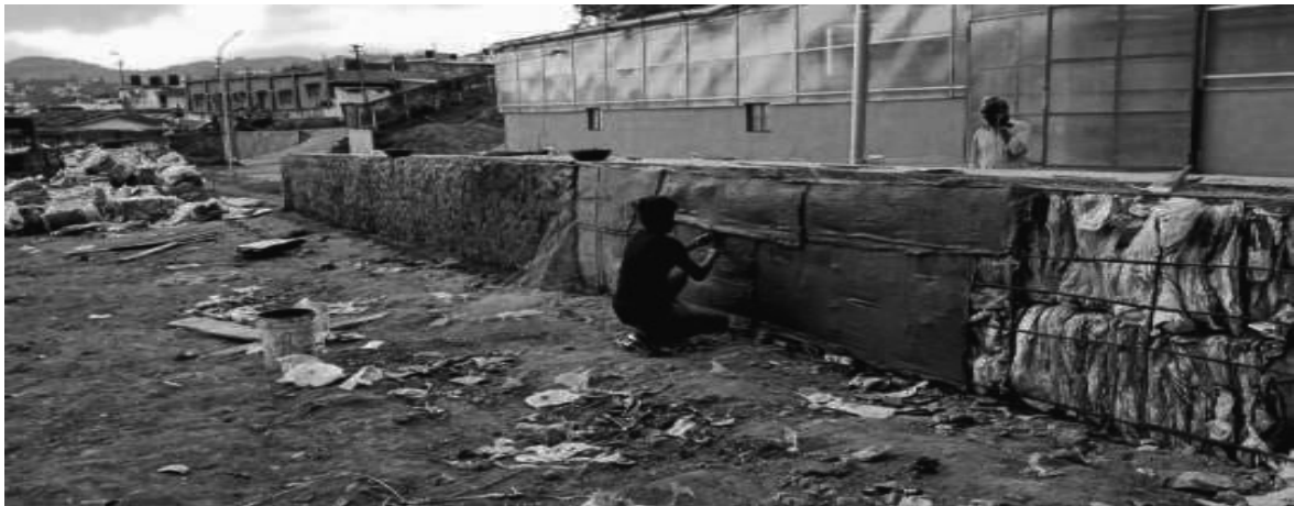
Construction of (Experimental) Plastic Retaining Wall at MICRO COMPOST CENTRE
