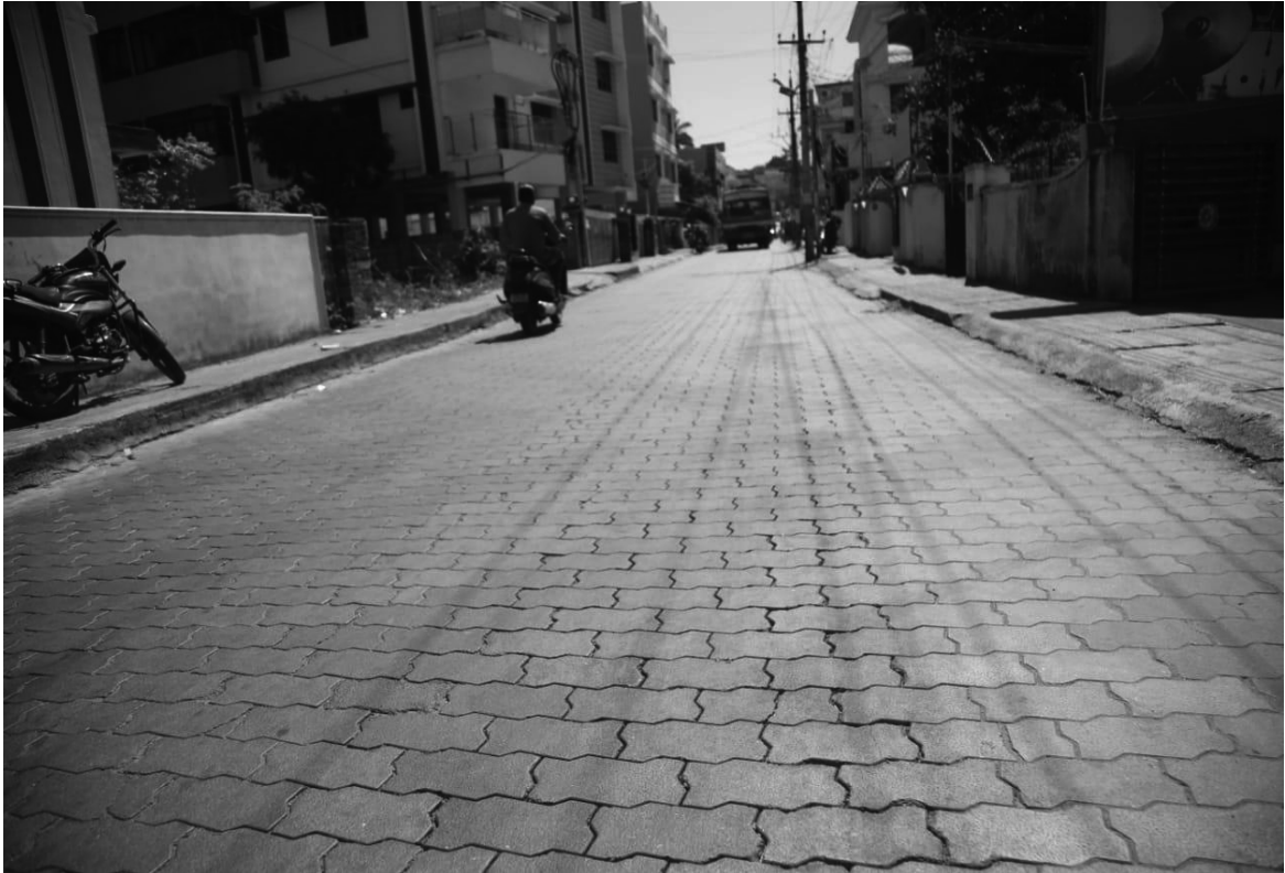
Paverblock road with cement concrete at the pavement in the street of Nagercoil
