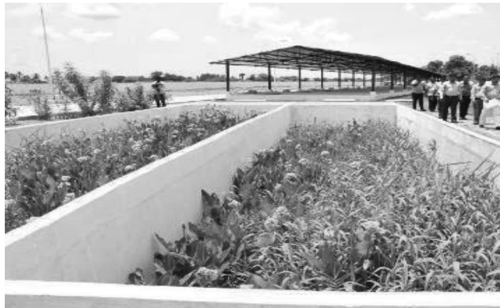
HORIZONTAL PLANTED GRAVEL FILTER (Size : 17.00x8.00m)
